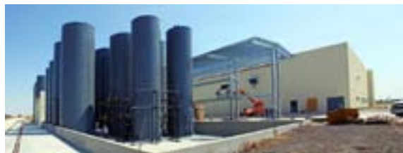
The Northland Oil facility is one of the newest Temple & Central Texas Railway customers.
