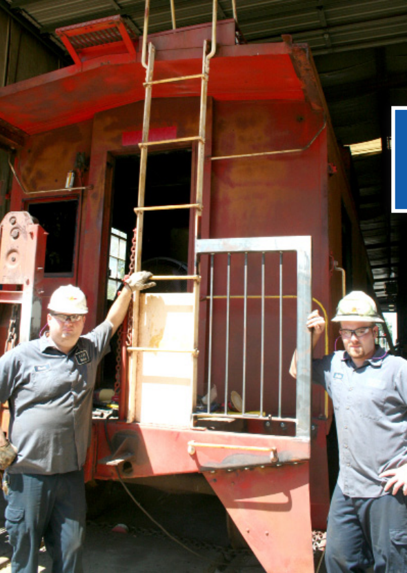
From left, Heath Harvey, electrician/machinist, and Justin Gorman, shop foreman, refurbish a caboose to be used for tours of LNW territory.
