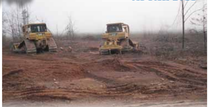
Bulldozers break ground on the Iron Bridge Road facility.
