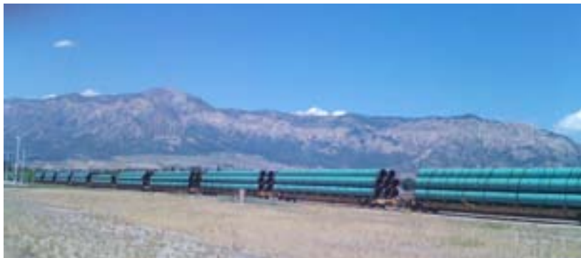
The months-long project brings multiple pipe shipments to Harrisville, Utah.
