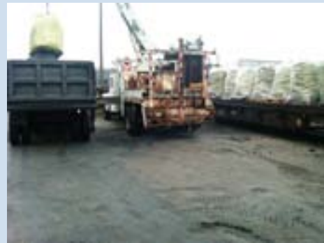
TSRR employees transload 2-ton bags of graphite from flatcars to a GrafTech dump truck.
